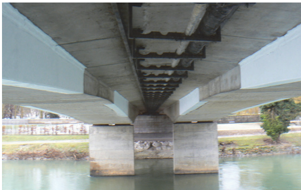
Fig. 17. View of the bridge under consideration; FRP repaired zones correspond to the white parts on the girders.
